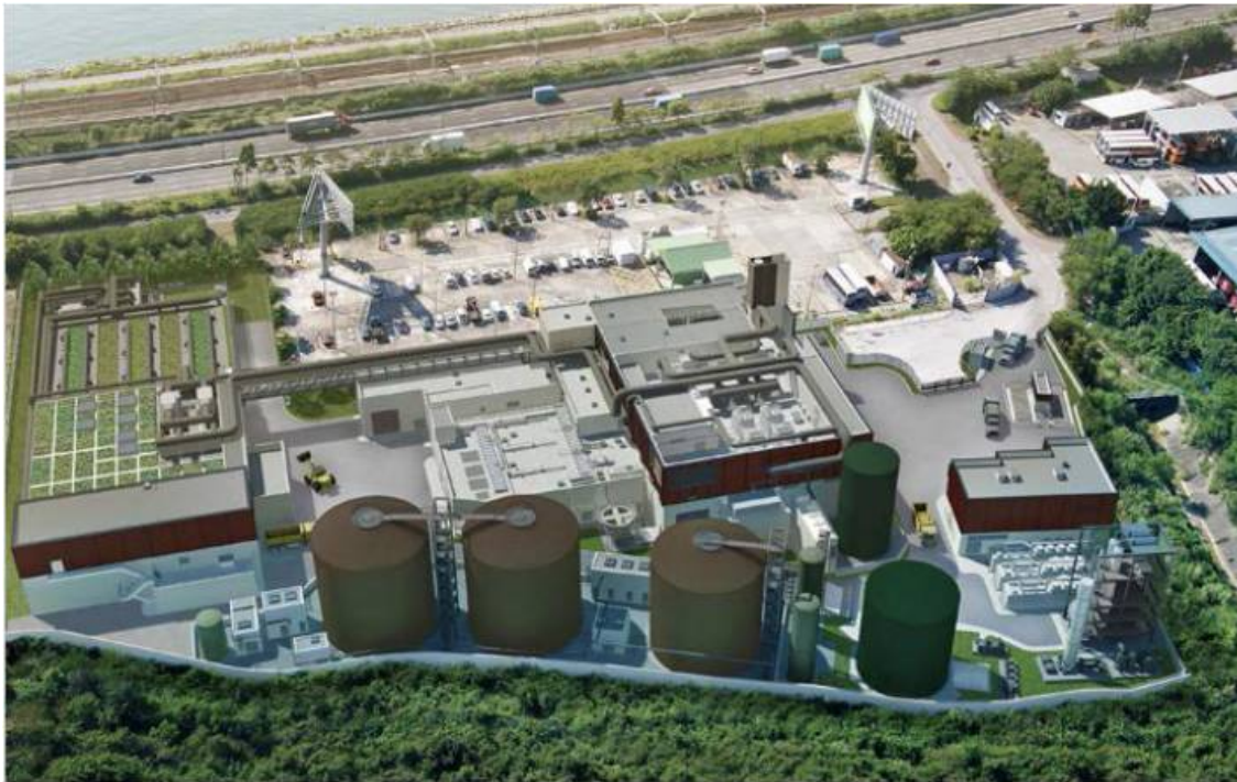
Source: Organic Resources Recovery Centre Phase 1 (OPARK1, previously known as ORRC1) image courtesy of Environmental Protection Department
